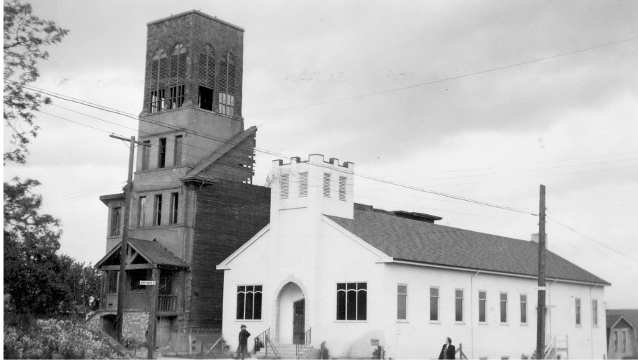
The new building in April 1954. Behind it is the partially demolished 1911 building. 22
